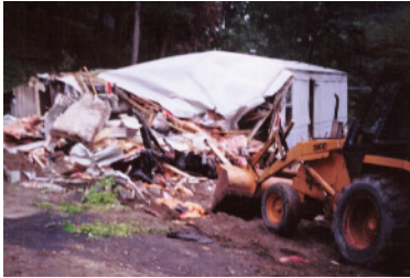
Mark demolishing the trailer
