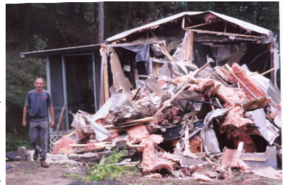
Mike Payne—demolition labor
